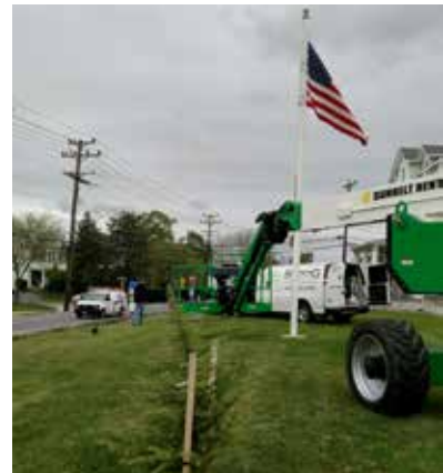
New flagpole installation at the Council Home
